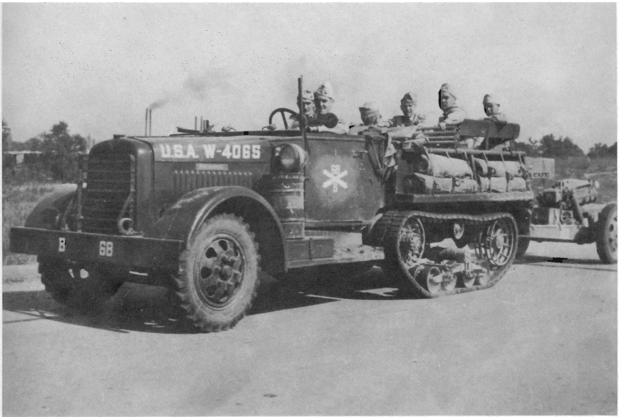
Ancestor of the armoured half-track was the T 5 artillery prime mover, like this vehicle of Battery B, 68th Field Artillery towing a 75mm M1A1 field howitzer.
