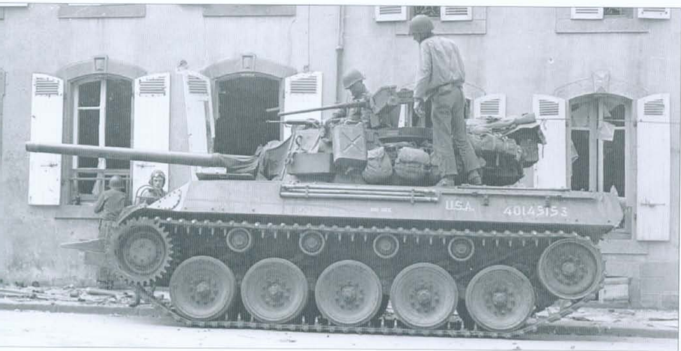
Two of the three M18 battalions of Patton's Third Army took part in the fighting for the port of Brest: this is "Big Gee" from the 1st Battalion, 705th Tank Destroyer Battalion which was supporting the 2nd Infantry Division during the fighting. It is from the second contract batch, accepted in February 1944. The set of "rhino" hedgerow cutters has been fitted to the tank. (NARA)
