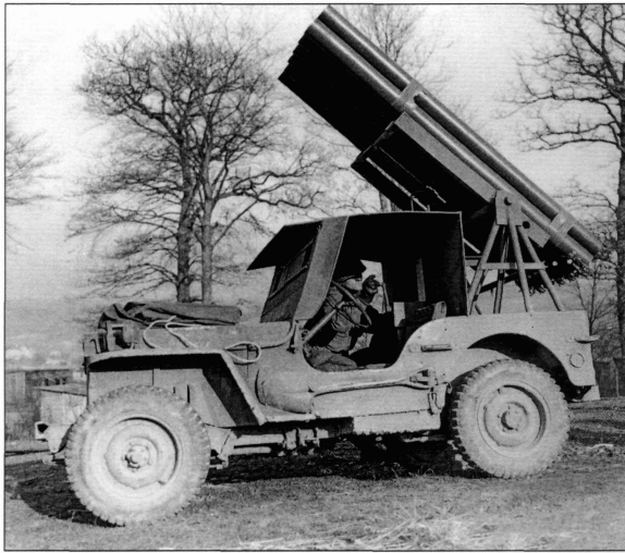
An ordnance unit in the US Seventh Army built a 4.5in rocket launcher on a jeep using M14 launch tubes designed for fitting on aircraft. This example is seen in action in Alsace in December 1944. (NARA)
