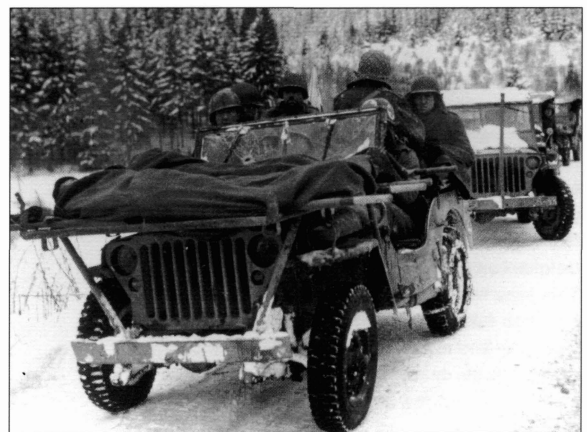
This jeep with the 334th Infantry, 84th Division during the Battle of the Bulge on January 9, 1945 shows a typical configuration with a frame over the hood to permit two litters to be carried on the front. (NARA)
